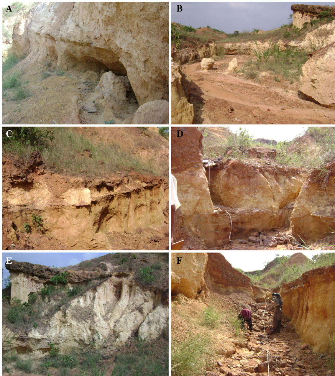
Fig. 8 Gully erosion processes in the Garbheta block. a Sidewall erosion, b gully widening, c active gully erosion during heavy rain events, d gully formed by retrogressive erosion with narrow and
