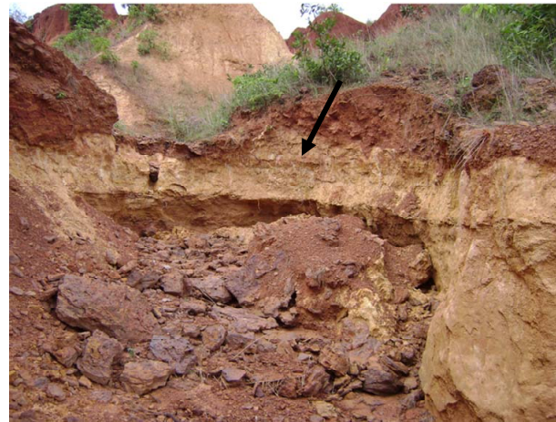
Figure 5. Collapsing the successively top bed rock in the gully head wall due to loss of cohesive force and under laying support, with the adding of moisture content.
